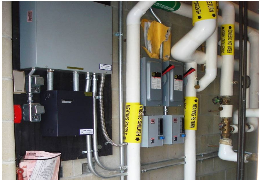
The Invensys LON-based Direct Digital Control (DDC) system was installed during the construction.
