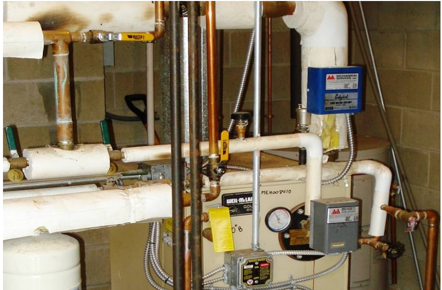
The Invensys LON-based Direct Digital Control (DDC) system was installed during the construction.
