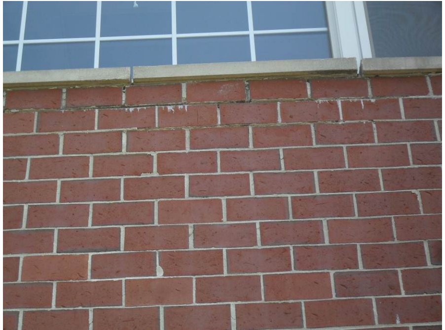
Second Floor Window Sill Damage
